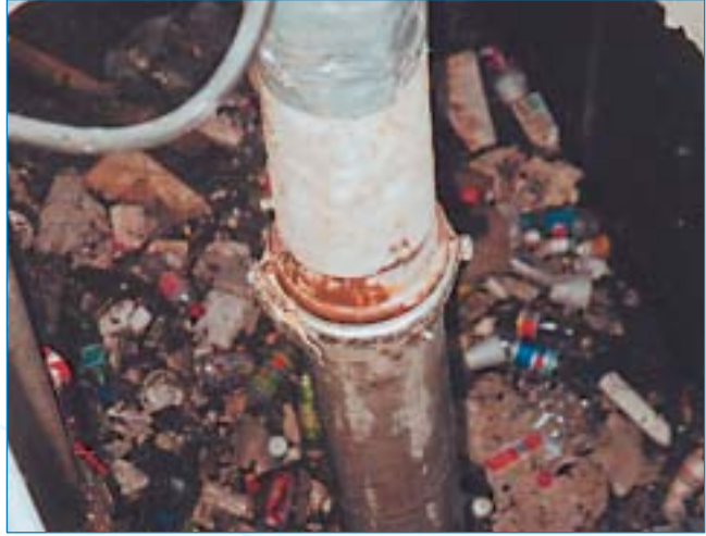
Captured and retained pollutants in the Ecosol RSF 4000 unit
