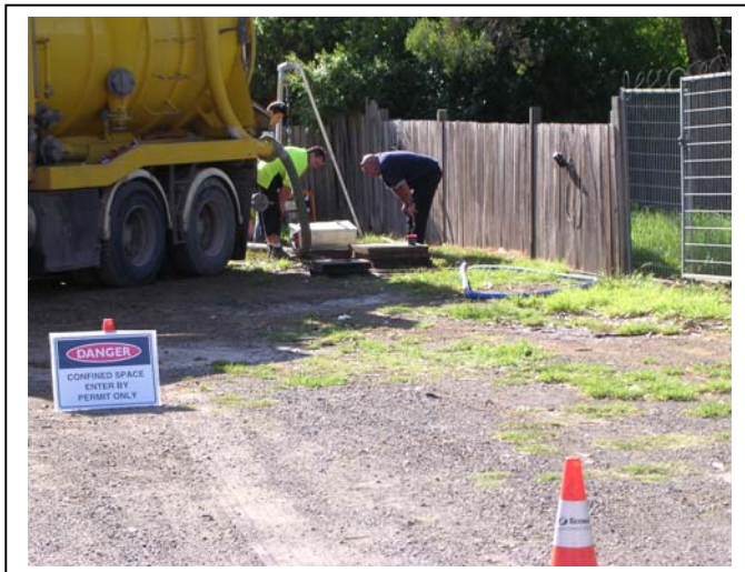
Inspection of the unit prior to cleaning
